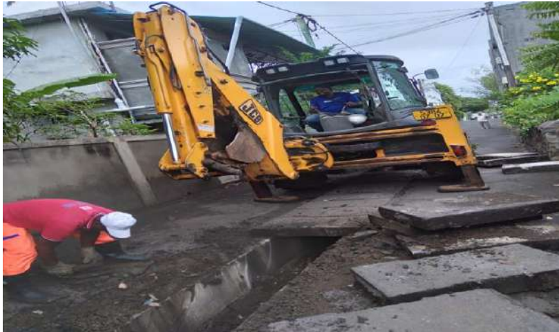
Cleaning of covered drain with excavator
