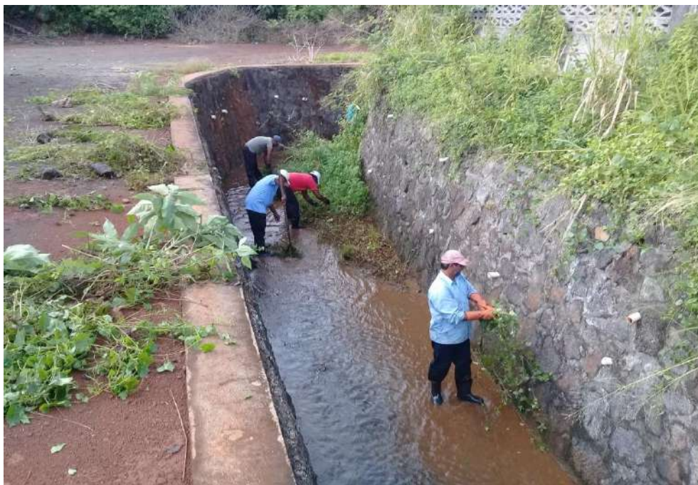
Cleaning of open drain manually
