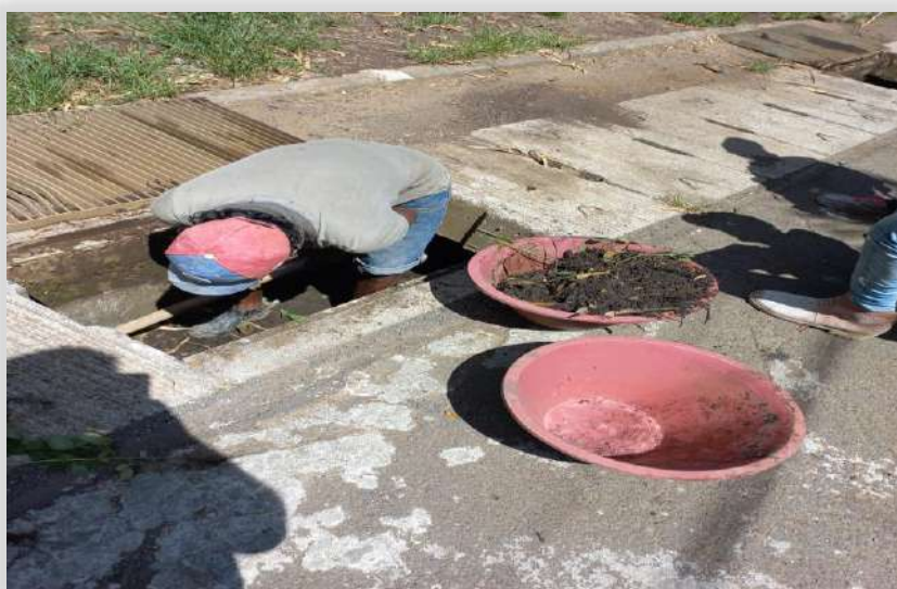
Cleaning of Covered drains
