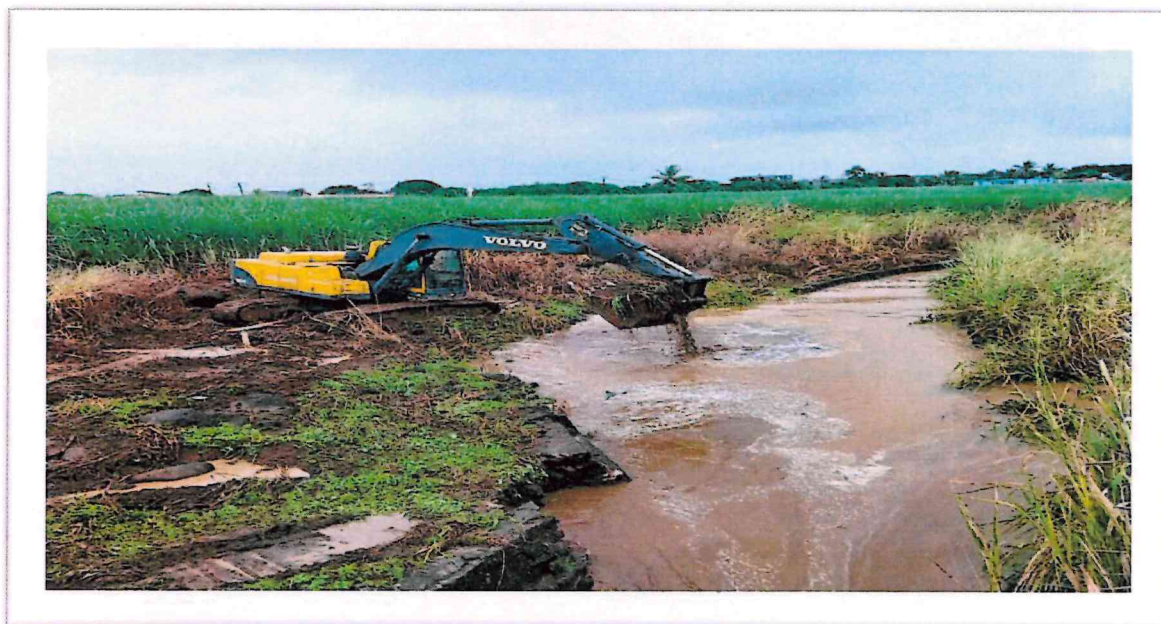
Mechanical Cleaning of open drain after heavy rain at Amitie
