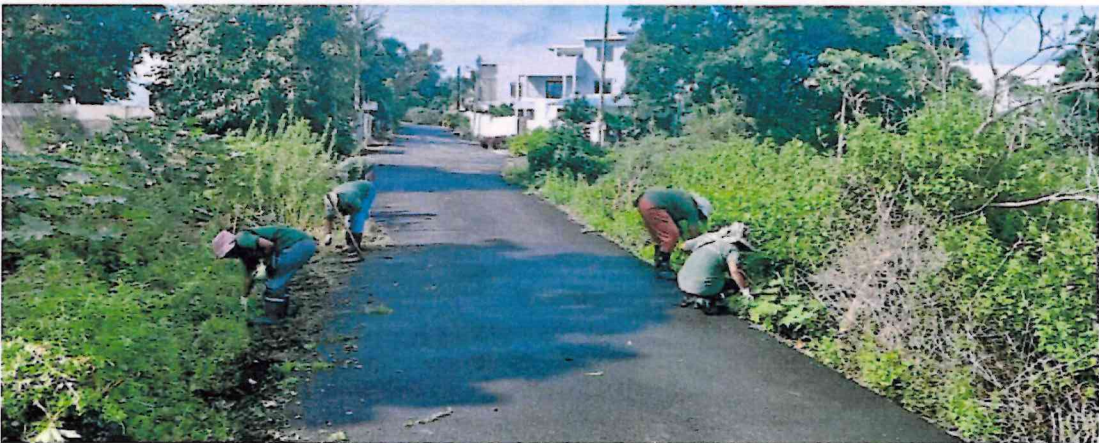
Mowing / weeding works along non-classified roads
