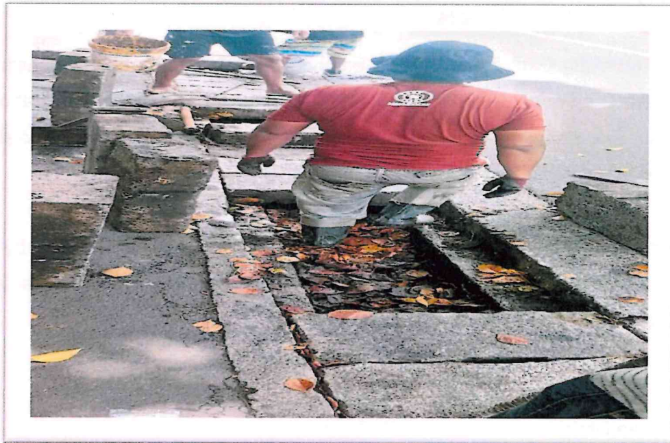
Cleaning of covered drain
