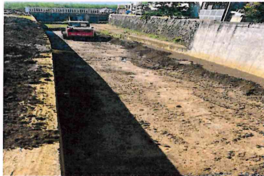
Cleaning of open drain at Gokhoola
